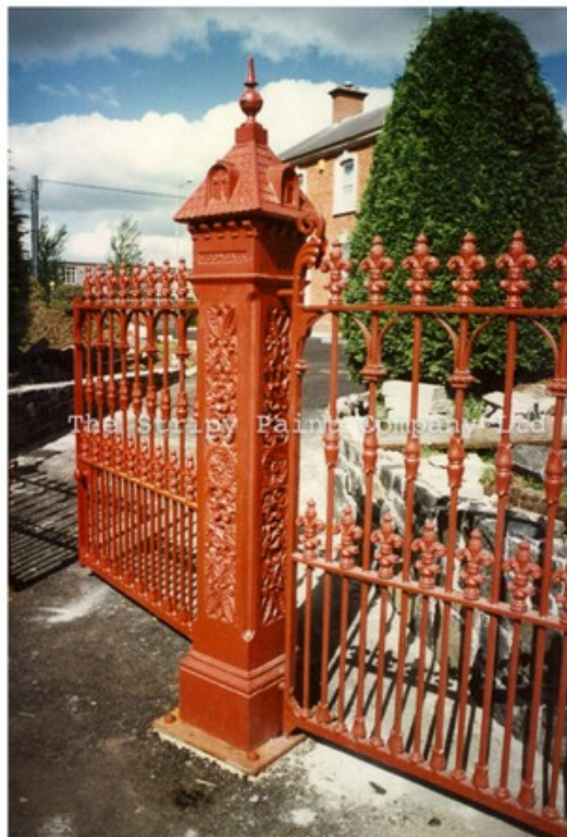
Cast Iron Gates And Gate Posts Made To Match Original Gates
