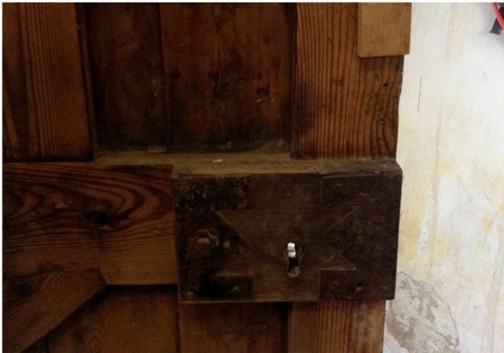
Wooden Rim Deadlock Made To Match Existing In Reclaimed Pitch Pine And Using Off The Shelf Rim Deadlock.
