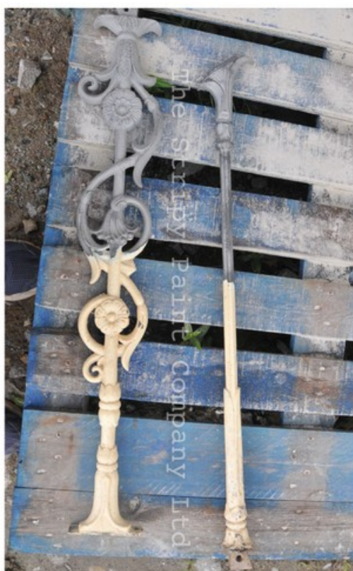
Extension To Existing Stairs Requiring New Cast Iron Balusters
