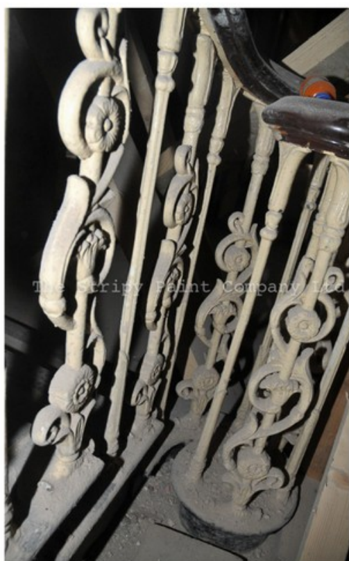
Extension To Existing Stairs Requiring New Cast Iron Balusters
